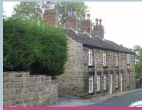
Coursed sandstone together with natural slate roofs, are the predominant materials of the conservation area.
