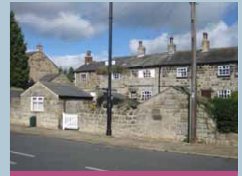
The historic development of Shadwell can be seen through the varying scales and types of historic building within the conservation area.
