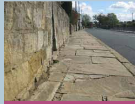
Coursed sandstone boundary walls and sandstone flags and kerbs make a positive contribution to the character and appearance of the conservation area.
