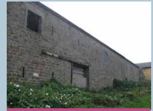
Historic farm structures add another layer of architectural types which add variation to character of the conservation area.
